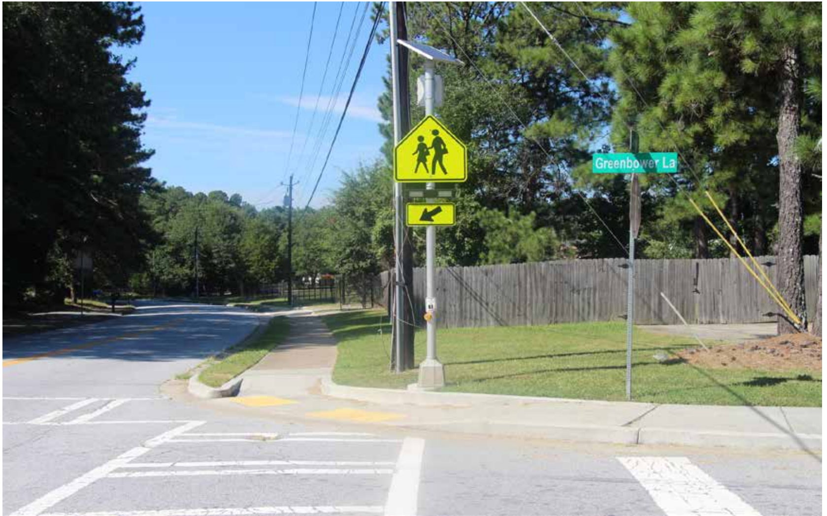
Rapid Flashing Beacons installed on walk routes
